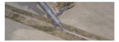
Depending on joint depth and the cracks associated with the joint – it is often necessary to add additional sand filling into the saw cut then set the backer rod in place. For additional strength – reinforced with fiber mesh joint tape.
