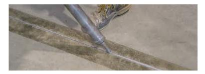
Depending on joint depth and the cracks associated with the joint – it is often necessary to add additional sand filling into the saw cut then set the backer rod in place. For additional strength – reinforced with fiber mesh joint tape.
